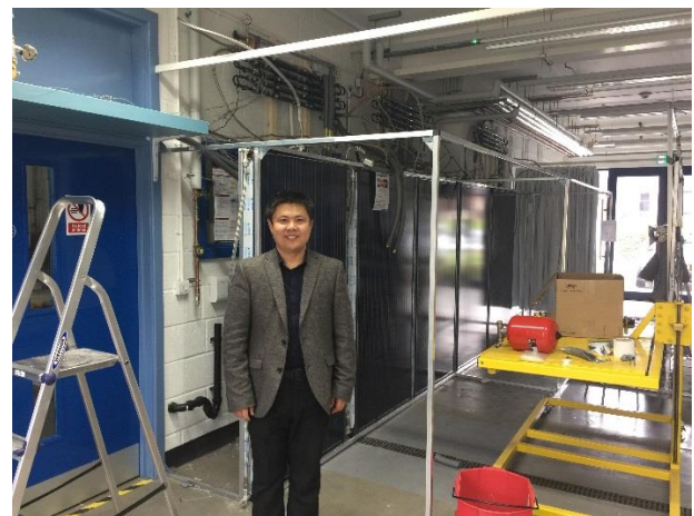
BIPV/T system at University of Hull.
